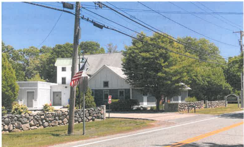
Many commercial property owners in Charlestown recognize its rural appeal. This commercial site has a harmonious relationship with its surroundings.
